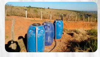
Just this filter itself is able to purify about 98% of water impurities. After this process, water goes through the **chlorinator**, nice scientific name, no? Well, this is nothing but a set of pipes and junctions in which we put chlorine pills. After water gets in touch with chlorine it's gets 100% pure and can be safely stored in the water tank, normally located in the house roof.
