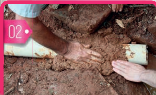
02. A two-meter-long pipe (6.56 ft) is set in spring bottom. This pipe is closed at its outer end and will only be opened in case it is necessary to clean the spring in the future;
