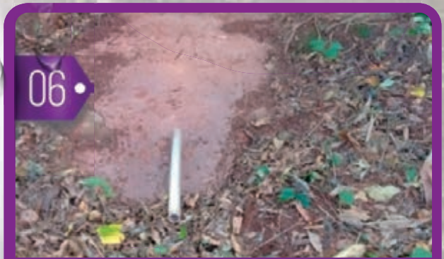
06. Finally, the whole spring is covered with a mixture of cement and soil so that it gets hard and protected.
